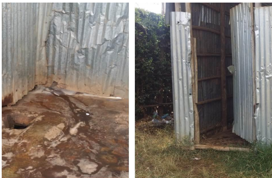
The current pit latrine at ET0167 – Fonko Kaleheywot Child Development
